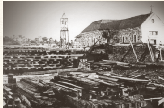
Local timber cut and prepared by workers for the monastery extension
